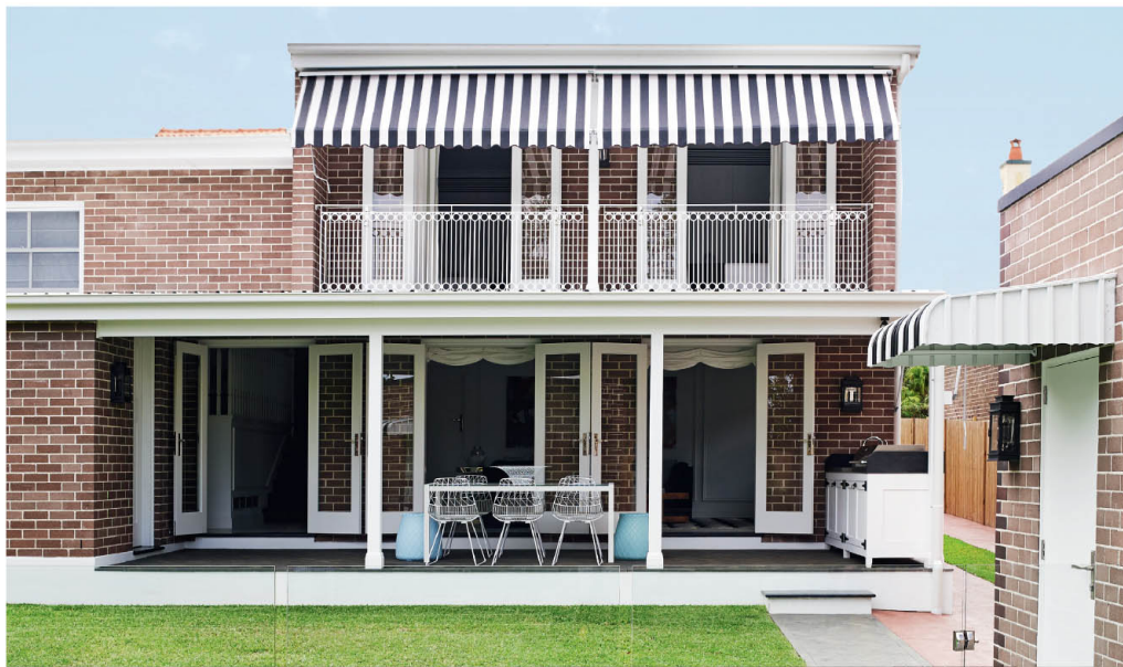
This page, clockwise from top the rear facade of the house was restored and the brickwork repointed. On the front porch, Loll Design Adirondack chairs from Own World. Tessellated floor tiles from Olde English Tiles Australia. In the kitchen a 'Bond' dining table from Jonathan Adler is matched with silver-leaf chairs from Regency Distribution. Visual Comfort 'Reed' pendant from Laura Kincaide. Ceramica Bardelli 'Architettura' tiles by Piero Fornasetti from Classic Ceramics. Vases from Melzai. Bowl from Space. Opposite page In the main bedroom is a Dorothy Draper 'Grand Lattice' bed from Kindel Furniture. Visual Comfort 'Ingrid' table lamp from Laura Kincaide. Greg Natale rug from Designer Rugs.
